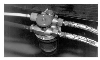
For pure single-pipe operation the bypass stopper must be unscrewed out of the return line opening and the return line opening must be sealed with a gasket and metal stopper.
